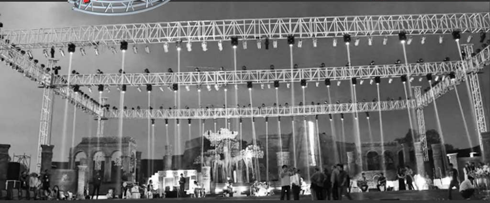
Actual site photograph of KWIK TRUSS installed at Madhya Pradesh Diwas by Phoenix Networks. Size 100 x 100 x 45 feet with 8 pillars.
