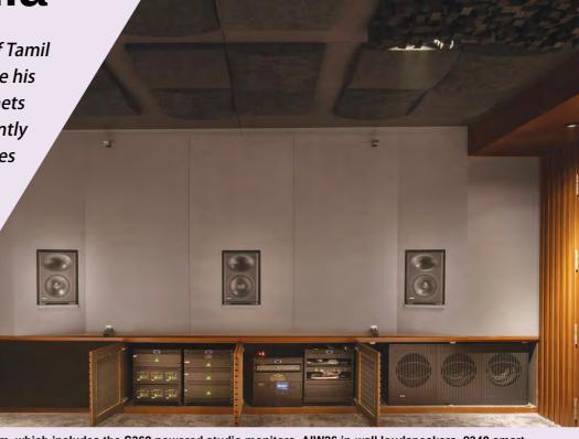
Genelec sound system, which includes the S360 powered studio monitors, AIW26 in-wall loudspeakers, 8340 smart active loudspeakers, and 7382 subwoofers, raise the acoustic quality of the plush home theatre in Southern India
