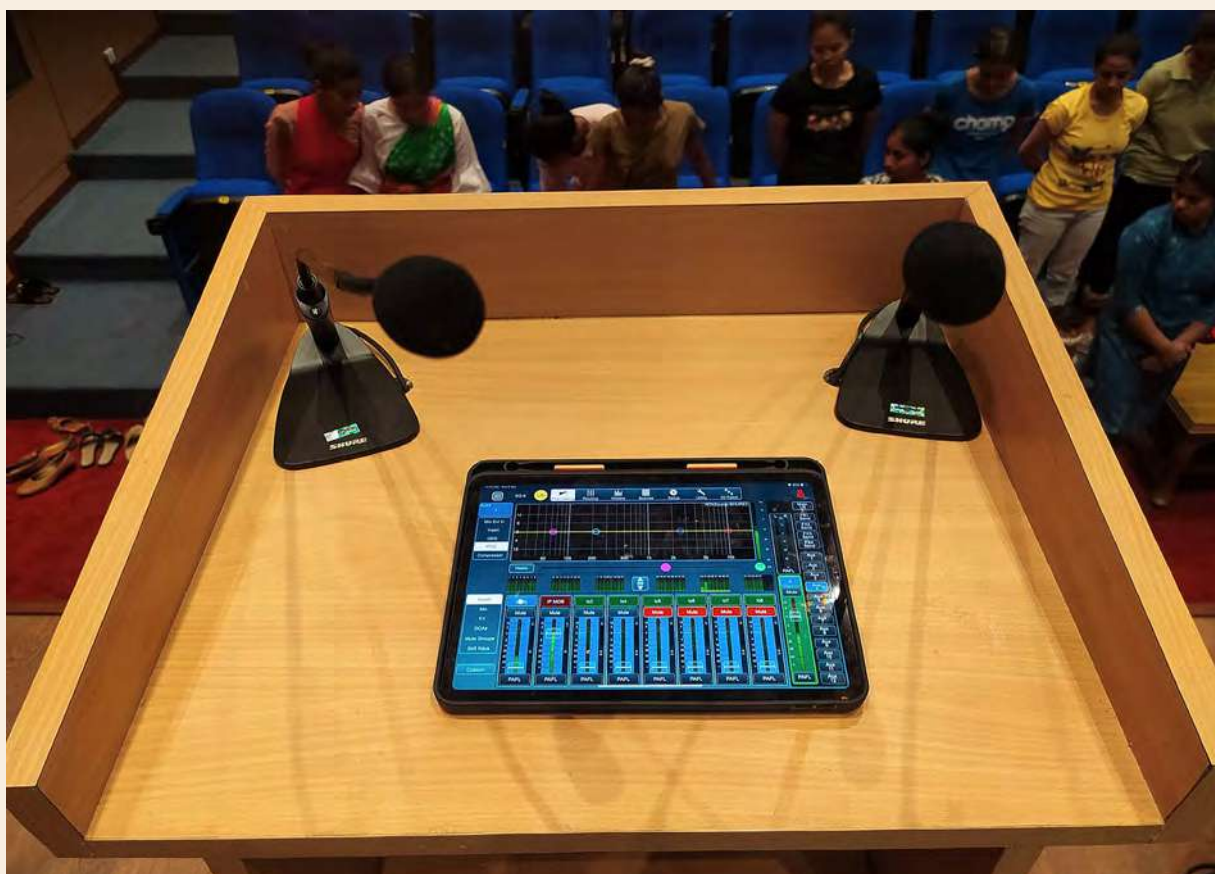
Shure Gooseneck microphones CVG12DRS-B/C have been installed on each of the two podiums on stage.
