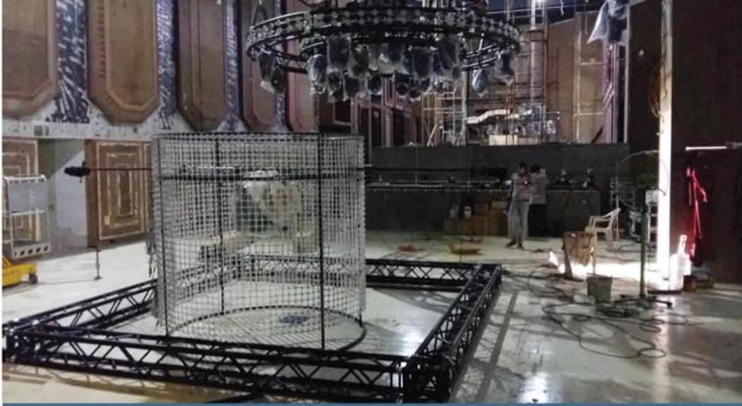
The central dance floor truss is shaped like a square with a cylindrical LED 50x50 pixel chandelier in it
