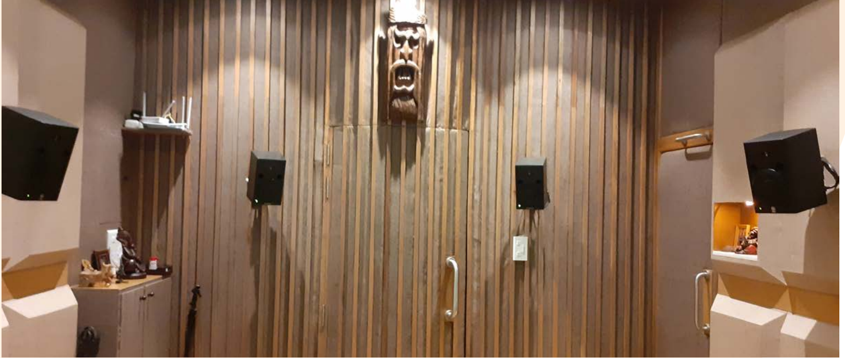
The entrance door on the back wall of Qfactor is curved - giving it a 'semi-cylindrical' shape. Double doors lined with magnets at the borders ensure that there are no gaps when the door closes.
